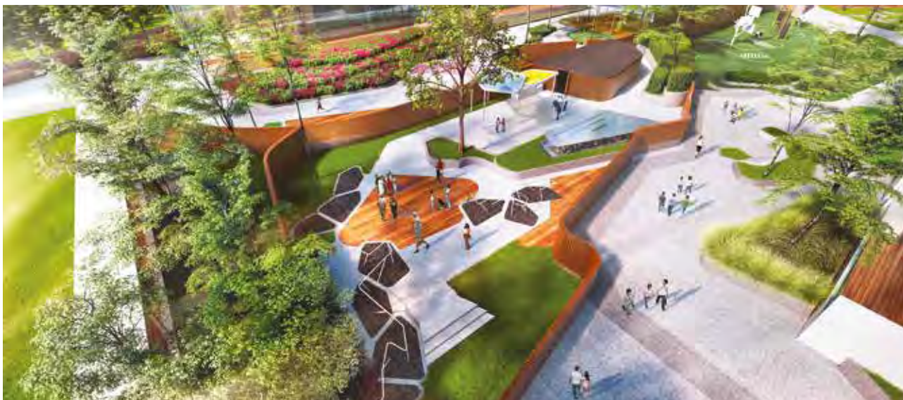
Facilities Area at Sunsuria Forum C-Suites, Setia Alam
